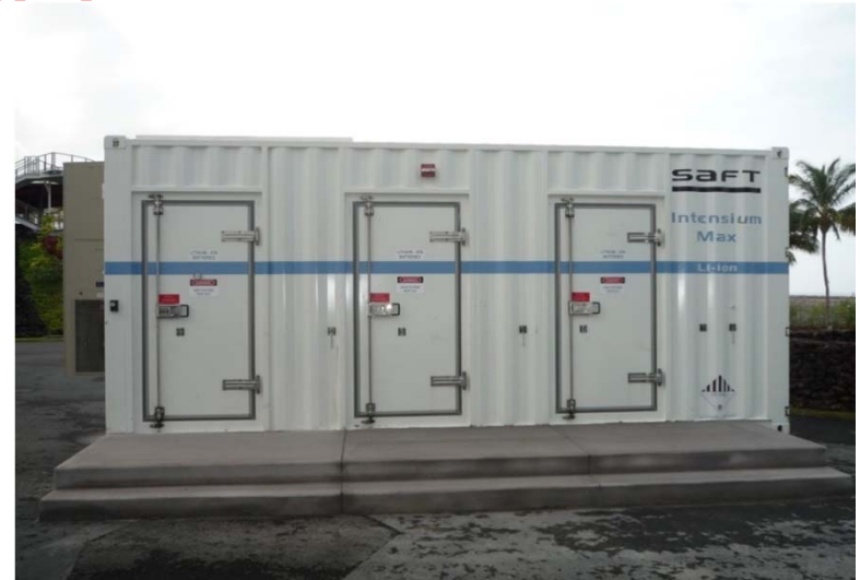
Lithium Ion Battery Installation – Koyo USA
