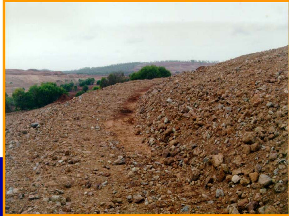
Dump 7 - Reprofile & Rock Line Outer Batters
