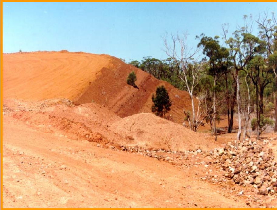
Dump 7 - Reprofile & Rock Line Outer Batters
